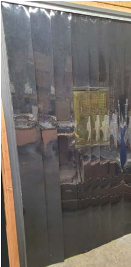
A black PVC curtain door with an amber window. Black gaffer tape attached to the outside of the door shuts off any cracks to prevent light entering
