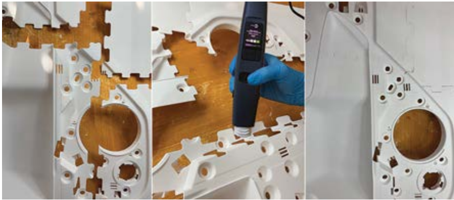
Pre-treating individual 3D printed parts prior to gluing them together with epoxy helps to establish a strong structural bond in the end product
