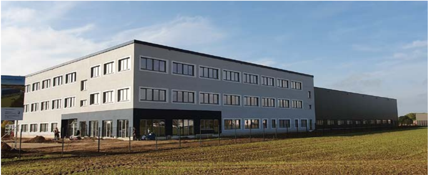
Continuous strong growth in all market segments over the past few years made it necessary for Koenig & Bauer Kammann to relocate to a new building with more space and customised facilities
