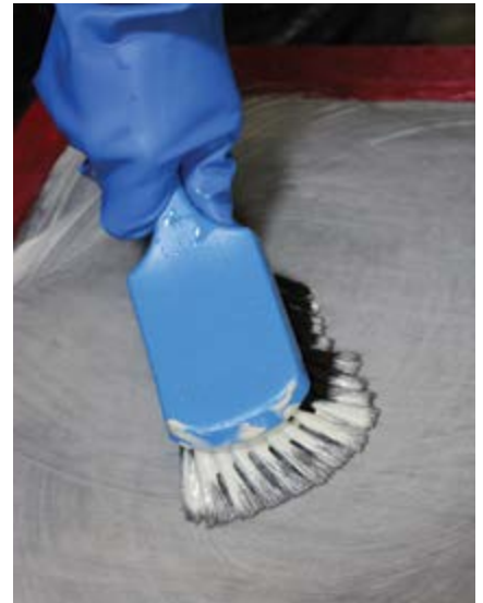
Use the special chemical brush to apply haze removers
