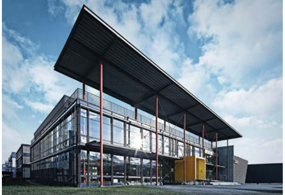
Zünd's headquarters in Allstätten, Switzerland
