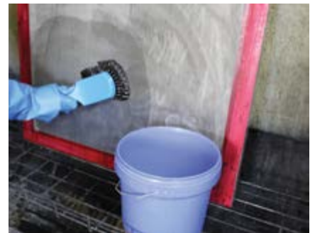
Use a chemically resistant brush to apply the haze remover
