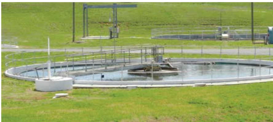
Settling of solid materials
