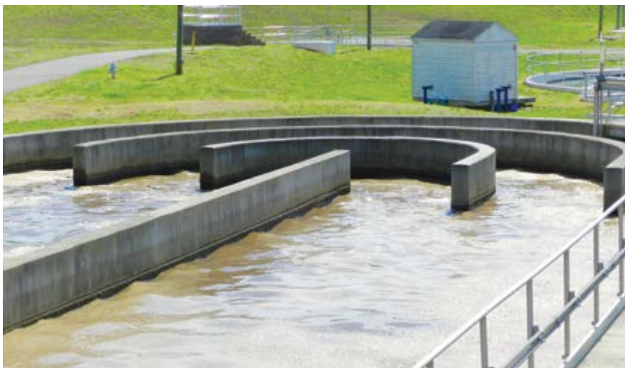
Constant aeration and agitation of sewage upon plant arrival
