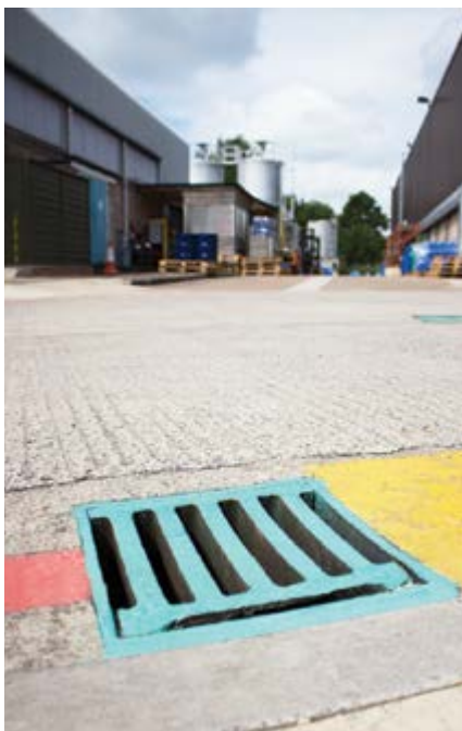
A top tip is to consider colour-coding your drains to identify between a domestic waste water drain and a trade effluent waste water drain
