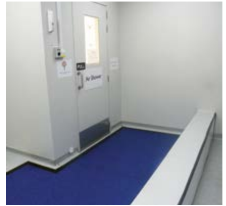
A final step over bench is used before entering the air shower
