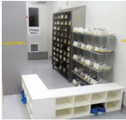
A step over bench is used when changing from outdoor wear to clean room overalls
