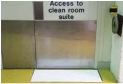
Tack mats are used as the first step in decontamination
