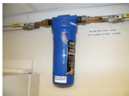
An in-line water filter will remove rust and limescale particles
