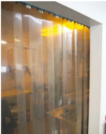
A vapour barrier doorway blocks mist or moisture from nearby sinks
