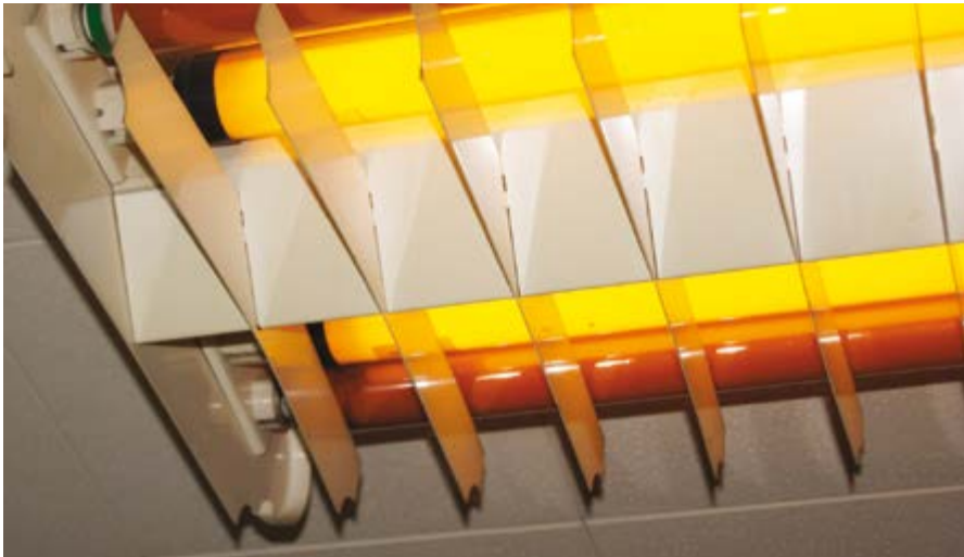
Yellow fluorescent safety lamps are needed in screen coating and storage areas
