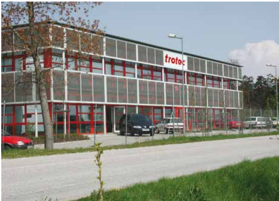
Trotec Laser's head-quarters in Wels, Upper Austria
