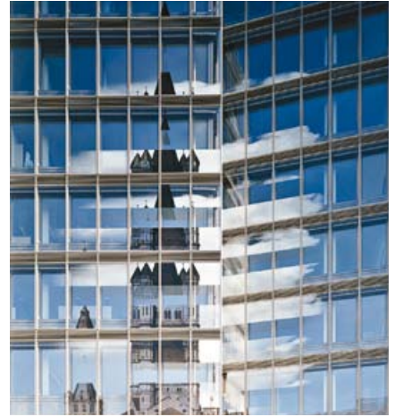
Printed architectural glass façade.
