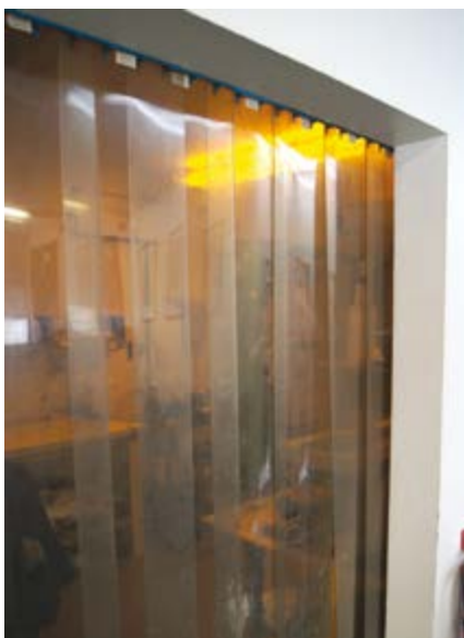
A multi panel plastic 'door' prevents outside air from entering the screen room
