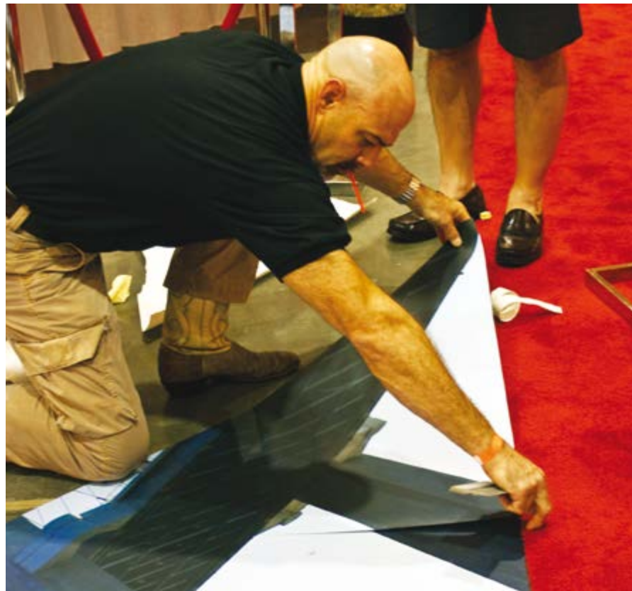
A removable adhesive allows for repositioning, if needed, during installation, as well as easy removability without damaging the floor when the graphic is no longer needed.
