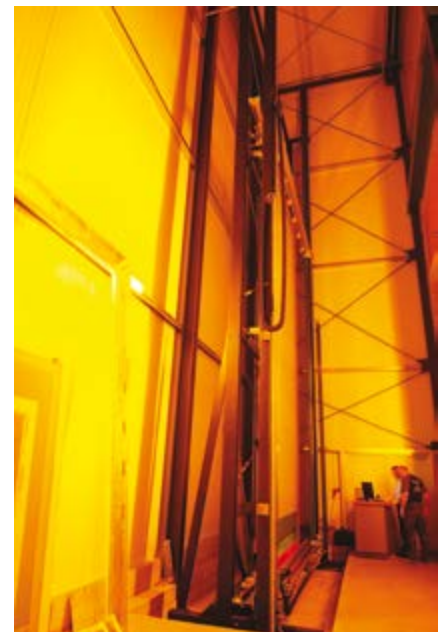
The installation is nearly finished
